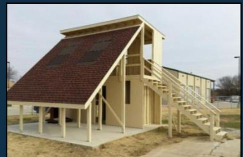
Phase I contains 10 different training props including: firefighter rescue/survival, forcible entry, ventilation, and ground and aerial ladder operations. Future plans include adding technical and vehicle rescue props.
