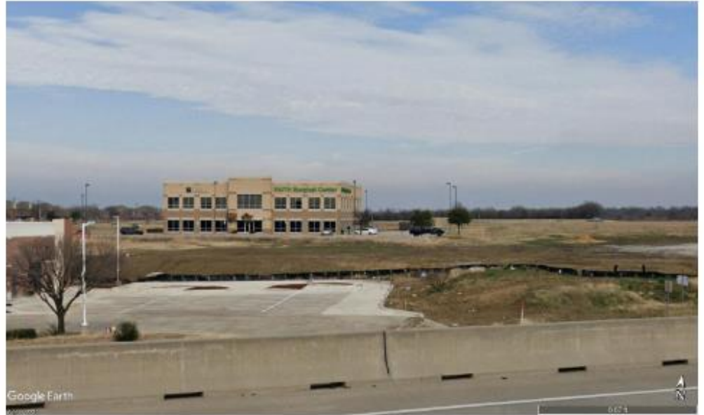
Southside Elevation from SH121 prior to new signage.
