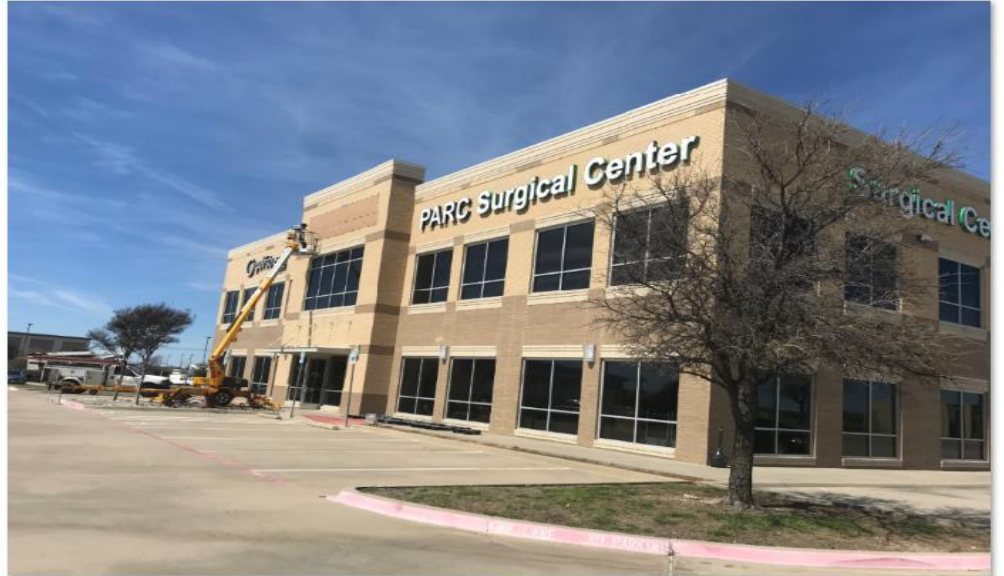
Southside Elevation during new signage installation.
